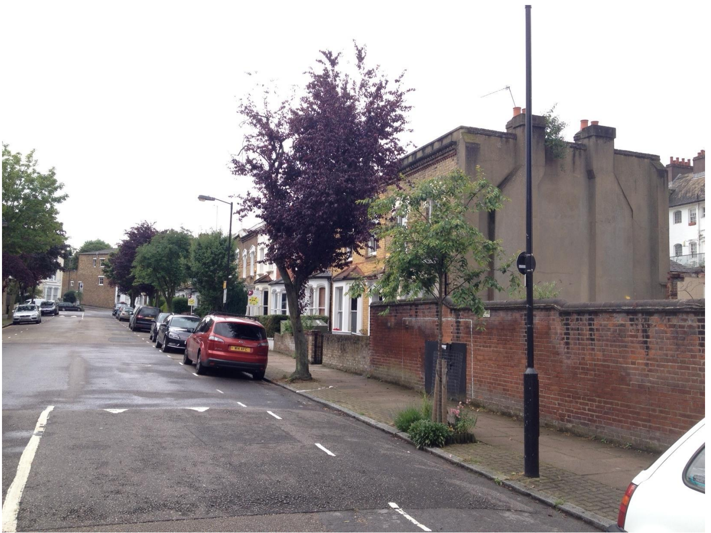
Photo 5 – Canning Road Terraces to south
